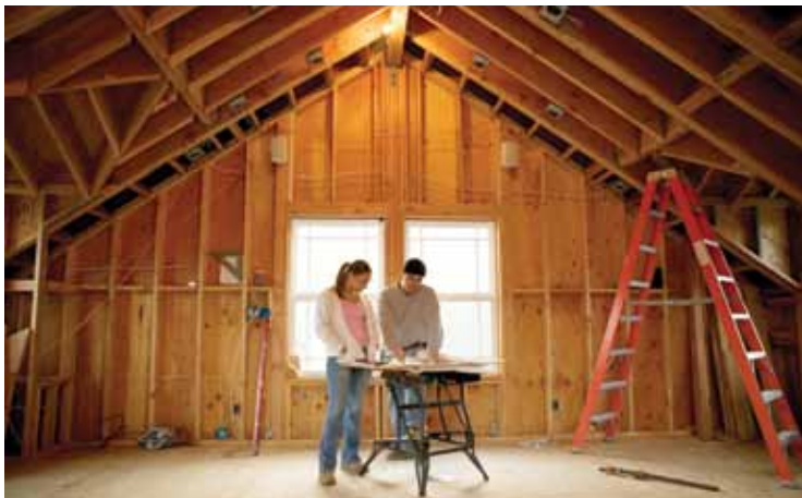
By installing a radiant barrier on the rafters in your attic, you can reduce the 140-degree temperature by about 30 degrees and save money.
