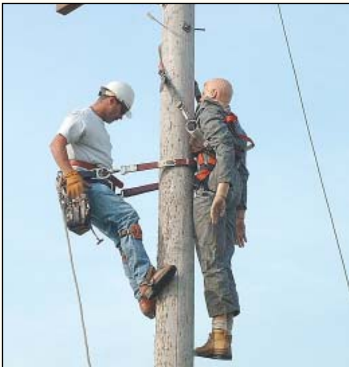
Henry Morrow, Lane-Scott lineman demonstrates the process of rescuing an unconscious lineman from on top of a pole simulated by a life-sized mannequin.
